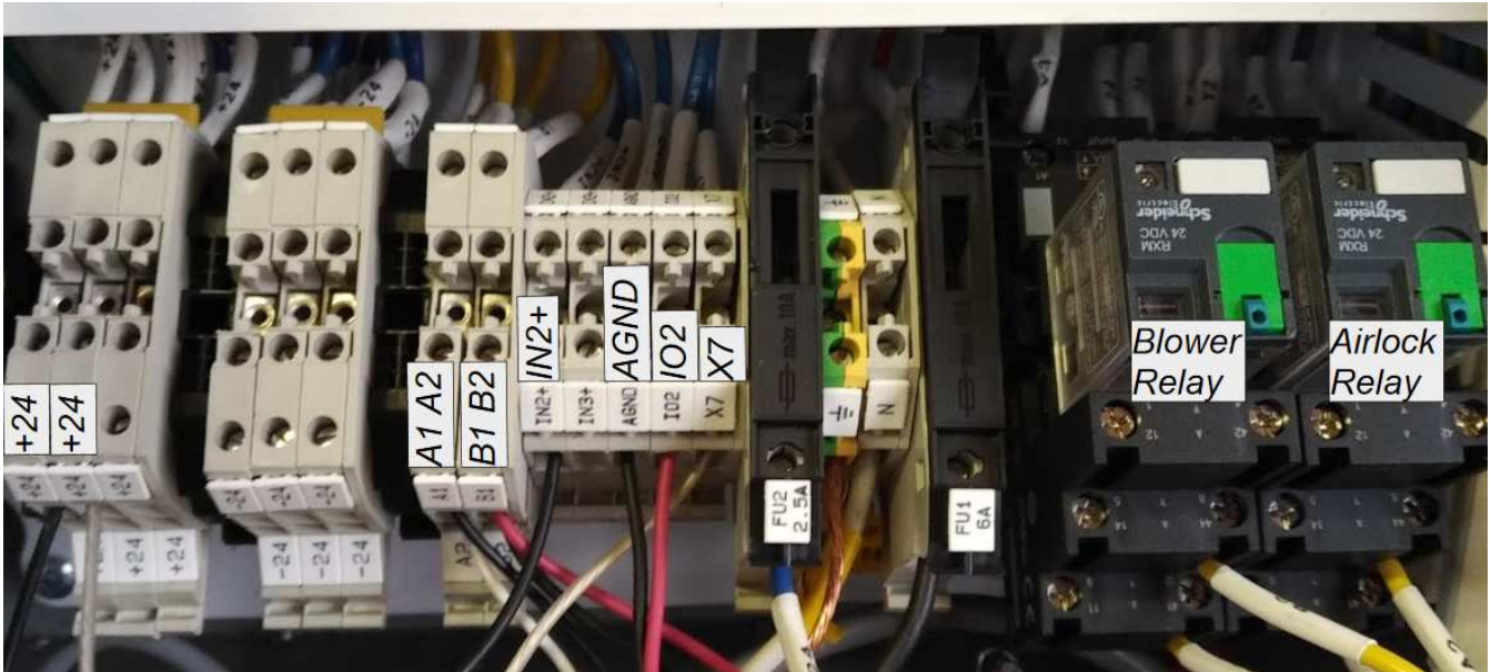
Figure 8 - PLC Wiring Module
